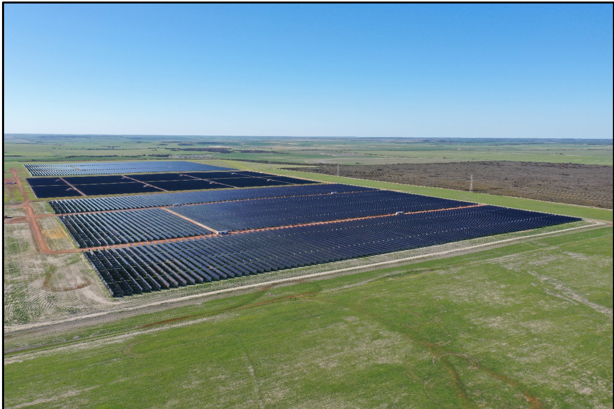
New stage 2 solar panels in the front and rear blocks with stage 1 panels visible in the middle
