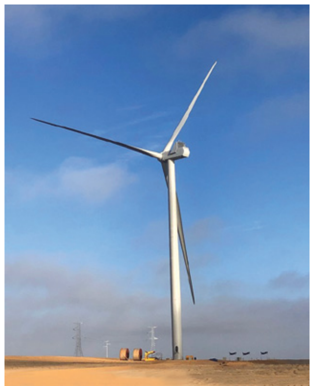
Pictured: The first erected turbine at the Warradarge Wind Farm.
